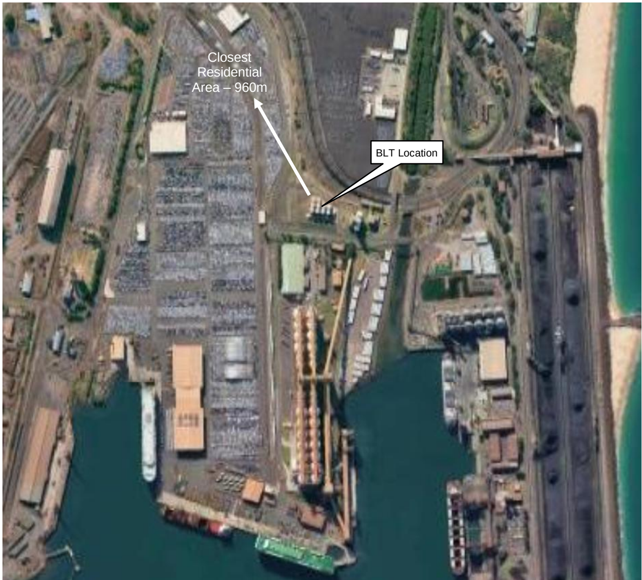
Figure 3.2: BLT Location in Port Kembla
